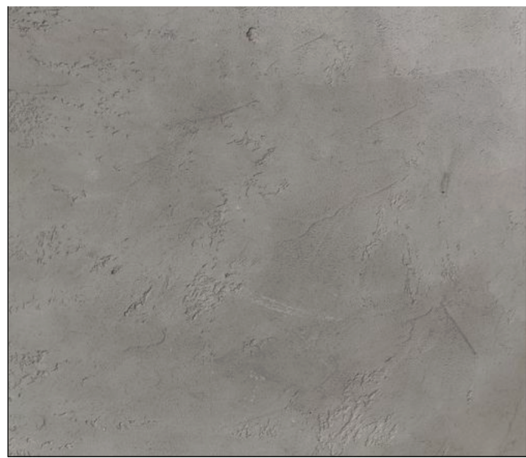
3 - LIGHT GREY CONCRETE FINISH - OFF-FORM CONCRETE
